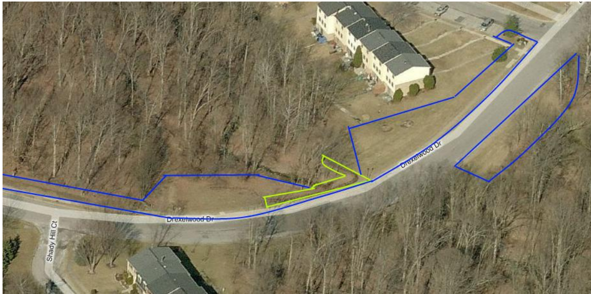
Figure 6: Drexel Woods Drive and the Culvert area
